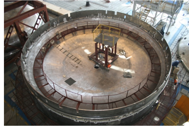
Mounting of the reactor vessel bottoms
